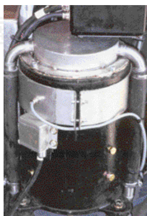
PUMP MOTOR IP 55 ENCLOSED
